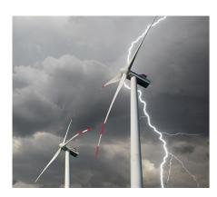
Due to their height and exposed location. wind turbines are especially susceptible to lightning strikes. A lightning protection system protects the rotor blades, bearings and gearboxes from lightning damage and prevents costly downtime caused by lightning
