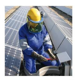
DEHN has developed an arc-fault-tested protective suit and jacket for use in switchgear installations as part of the personal protective equipment. In combination with a safety helmet and gloves, protective suits and jackets for use in switchgear installations the risk of injury resulting from the thermal effects of arc faults during work on electrical installations is thus reduced.
