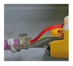
tems used e.g. for data acquisition and monitoring of PV systems it is advisable to use an EMC spring terminal for low-impedance contact with cable shields over large areas.
